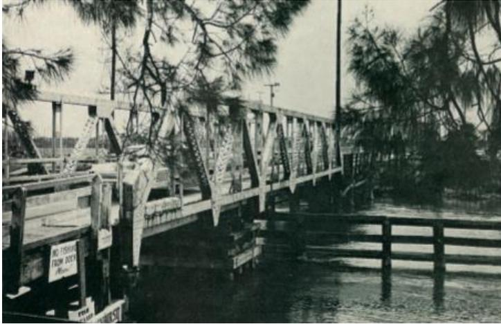
“PICTURESQUELY FRAMED by low-hanging pine limbs, the old Haulover Canal Bridge is more scenic than practical, and will give way next year to a new bridge now under construction. This one lane, wooden structure has been in use for more than 40 years.”
