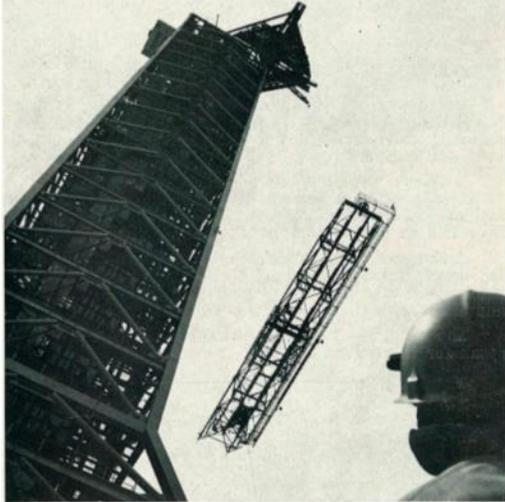
“A PROUD IRON WORKER watches the last major piece of steel, a 21-ton crane boom, hoisted up Launcher Umbilical Tower number one at Merritt Island. It was fitted into place at 2 p.m. Tuesday, topping out the steel work on the towering LUT.”
