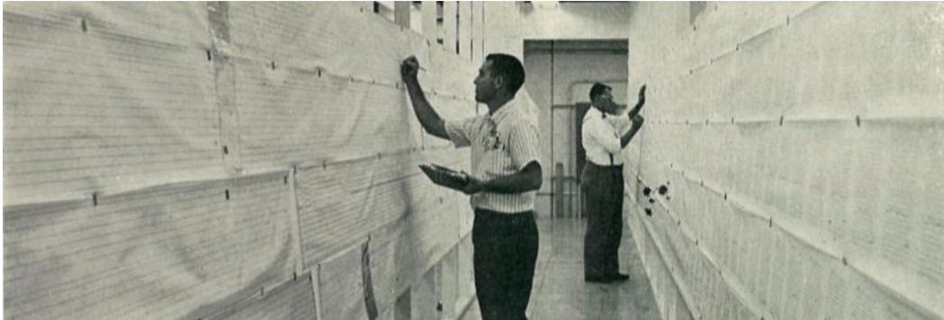
“FOR MANY PEOPLE at the Kennedy Space Center, the real work begins after a successful launch. Here, Bob Cessac, left, of the Calibration Control Section, and M. E. Carpenter of Chrysler, glean data from 147 telemetry oscillograms recorded during the recent SA-7 flight. Information gained includes temperature and pressure probes of the in-flight vehicle and control measurements radioed back to Earth. If laid end to end, the oscillograms would stretch for nearly half a mile.”
