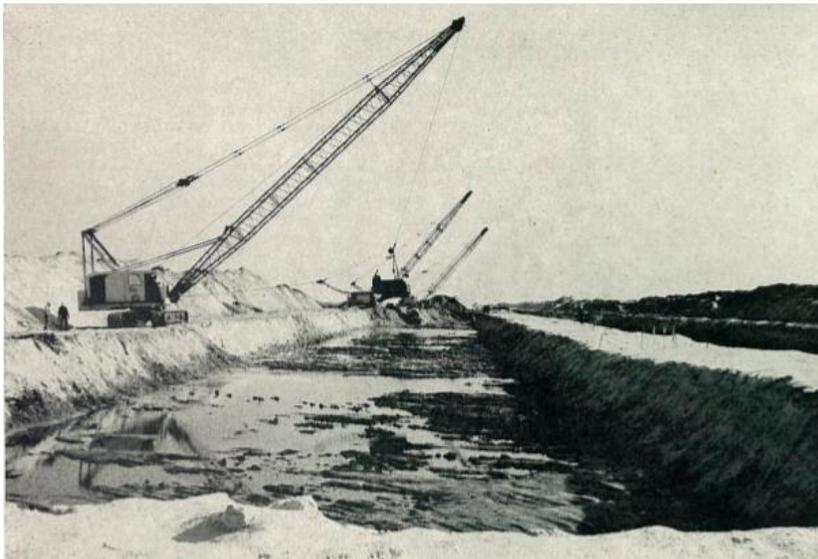
"DREDGES swing into action on the crawlerway between Complex 39's Pad A and the Vertical Assembly Building site. They are scooping out a "soupy-like" layer of Earth, which will be replaced with more substantial material."
