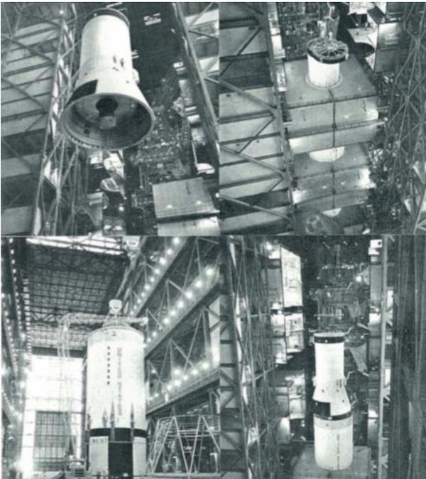
"STACKING OF the Saturn V launch vehicle for Apollo 15, to be launched next summer, was recently completed in the VAB. The second stage, lower left, was erected atop the first stage, and the third stage, upper left, and lower right, was then placed on the second stage. This was followed by placing the instrument unit on top of the third stage, upper right."
