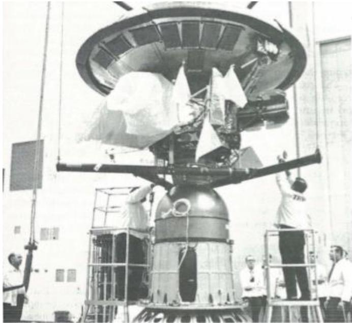
“ENGINEERS ARE performing a mating check between the Pioneer F spacecraft top, and a dummy third stage engine in KSC’s Hangar AO, Cape Kennedy. Pioneer F is scheduled for launch from Complex 36 on February 27.”
