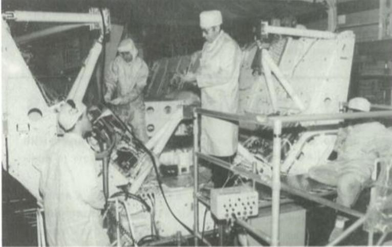
“ENGINEERS prepare pallet 1 on the Spacelab 2 payload for functional testing of experiments. From left are Mark Beaudreaux, Gerry Rivera and .Herb Brown, lead of the Networks and Power Group, Experiments Data Section.”
