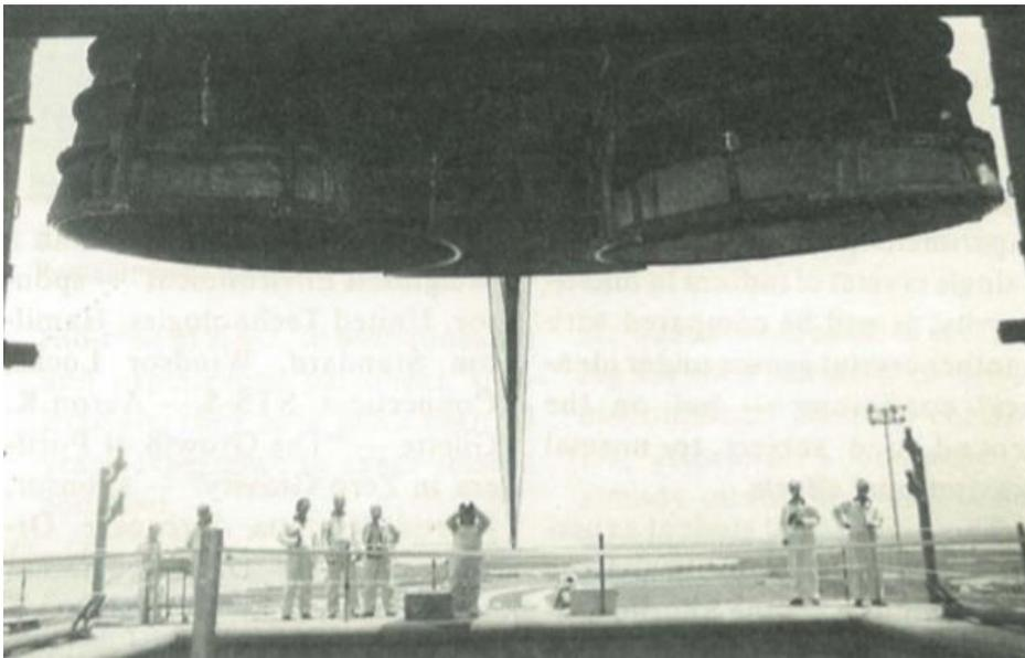
“INSPECTION TEAM members conduct an initial examination of the nozzles of Orbiter Discovery's main engines following the Mission 41-D abort.”
