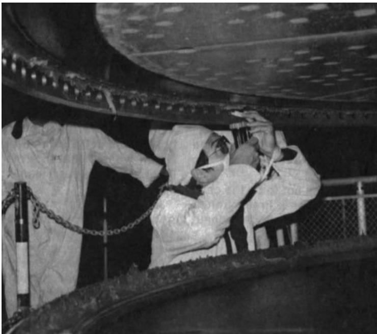
“TWO SEGMENTS of the left-hand booster, originally slated for space shuttle mission 61-G, are separated in the VAB. Destack operations on the left hand booster have been completed, and destacking at the right hand booster is in progress.”
