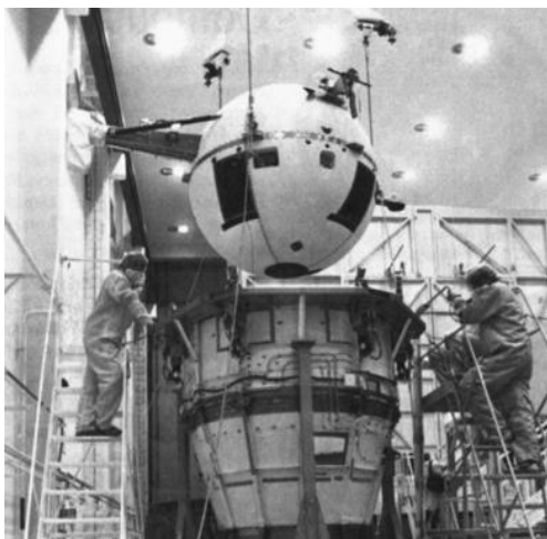
“AERITALIA AND MARTIN MARIETTA employees check the fit of the Tethered Satellite System satellite (TSS) with the satellite support assembly in the Operations and Checkout Building. The satellite is a cooperative U.S./Italian program scheduled to fly on Mission STS-46 in 1992.
