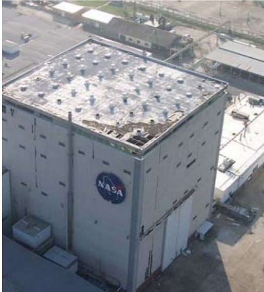
"ROOF DAMAGE to the Vertical Assembly Building..., above left , at the Michoud Assembly Facility. Right... is an aerial view of the damage to the External Tank Manufacturing Building at Michoud."
