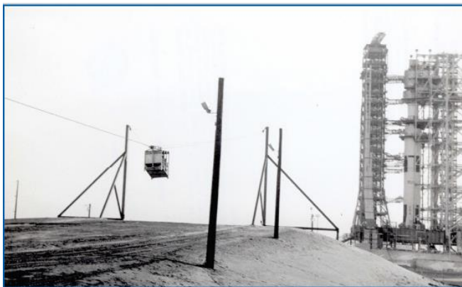
“The cab used for emergency egress from the Apollo/Saturn V rocket hits a reverse pull arrestor cable system which slowed it to a stop during the first manned run of the system from Launch Complex 39's Pad A on Jan. 25, 1969. Riding in the nine-person-capacity cab were astronaut Stuart Roosa, a member of the Apollo 9 support crew; Chuck Billings, KSC Safety Office; and Art Porcher, Design Engineering. In the background is the Saturn V launch vehicle for the Apollo 9 mission...”.
